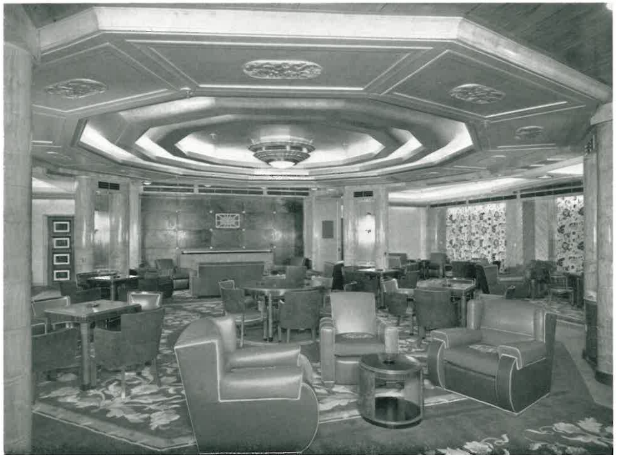
Architects and lighting engineers combined their experience to provide Caronia's lounges with illumination which is both efficient and in keeping with their dignified appearance. This moulded ceiling, which conceals fluorescent lamps above each of its sections, is one result of the partnership in design and lighting.
